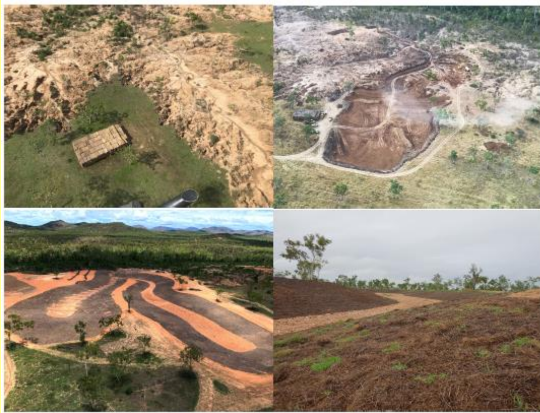
Figure 10. Selection of photographs showing the Strathalbyn gullies in various stages of construction: before (top left), during (top right) and after (bottom). Source: Brooks et al., (2020). Photo credits: top, D. Telfer; bottom, A. Brooks.
